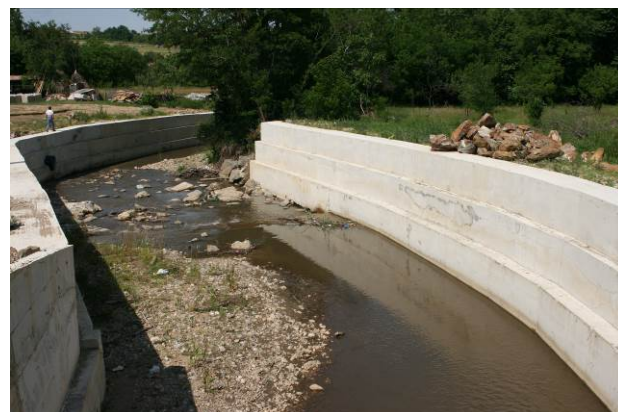
Fig. 5 Barcău river – Concrete river bed at Suplac
