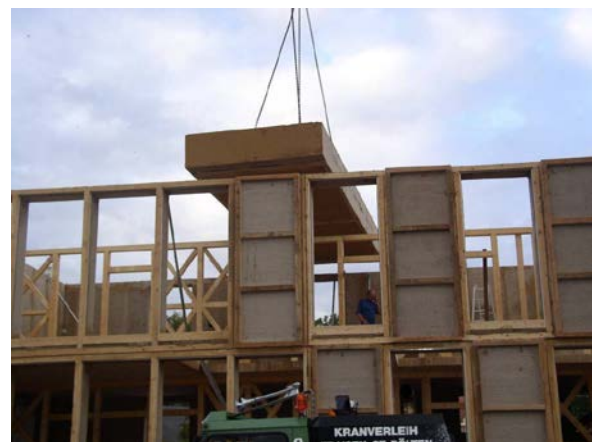
Fig. 2d Strawbale house in Tattendorf made of prefabricated blocks
