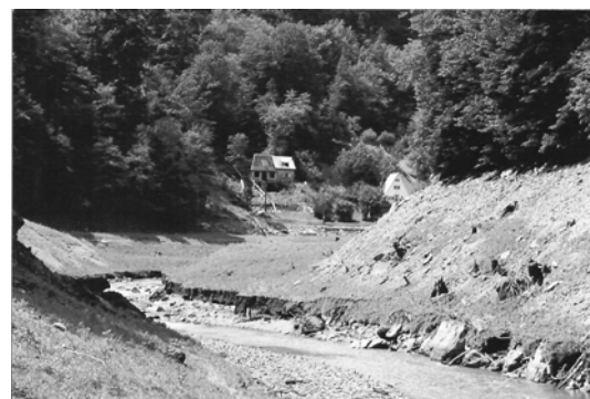
Fig. 9. The sediments deposits from Tarnița basin on the Someșul Cald branch. The thickness grow from the end of the retention towards the interior (0.30 m to 115 m and 1.21 m to 450 m distance) than they slowly reduce until the Someșul Rece II aqueduct outlet
